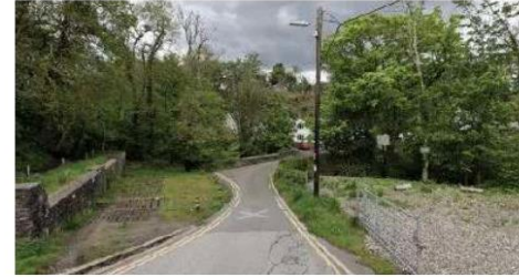
6 'accessible' parking spaces are located next to the entrance to the Waterfall Trail, but these spaces are not compliant with regulations
